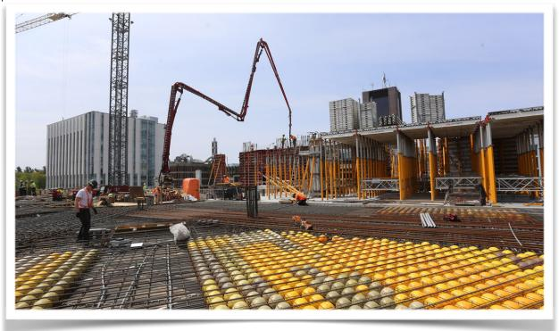
A total of 11,300 bubbles were used, displacing nearly 163 tonnes of concrete, with every kilogram of recycled plastic replacing roughly 100 kilograms of concrete.
